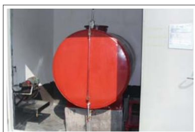
Fuel tank placed above ground
