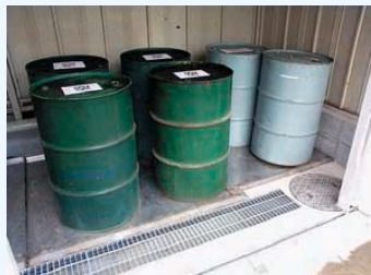
Grated pits around the place to keep waste water and containers for emergency
