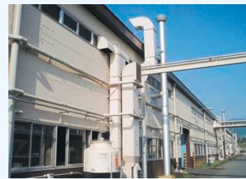
Visible plumbing (not in the ground)
