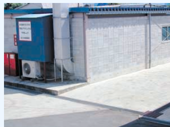
Grated pits around the dangerous substance warehouse
