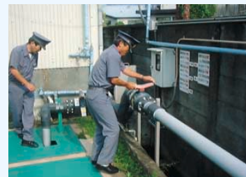
Emergency cut-off training for final discharge outlet
