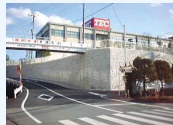
Repaired stone fence adjacent to public road
