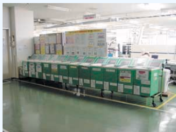
How to separate wastes and where to store them are indicated in both Japanese and English. This encourages personnel from the overseas subsidiary companies to cooperate in waste separation.
