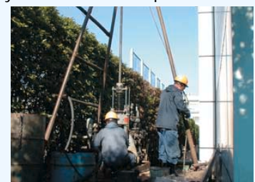
Digging for monitoring well
