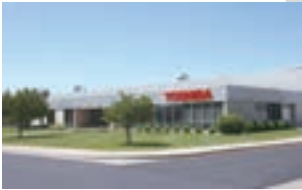
12 Toshiba America Business Solutions, Inc. (Plant)
