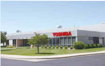
12 Toshiba America Business Solutions, Inc. (Plant)
