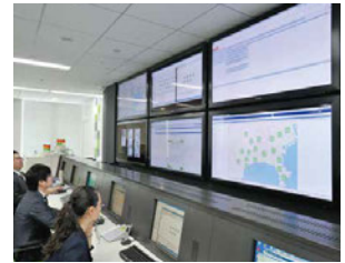
System support center
