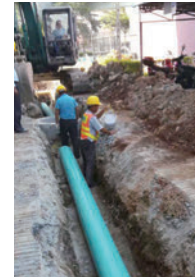
Toshiba Tec Information Systems (Shenzhen) Co., Ltd. Water pipe leakage prevention construction
