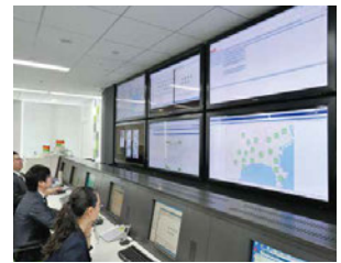
System support center
